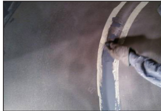
Applying ARC 858 to the weld seams
